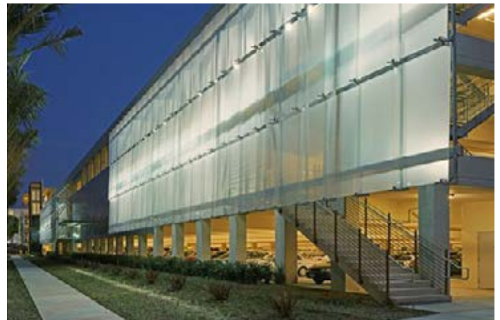
Structured parking incorporating upgraded materials
