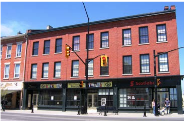
Consistent rooflines contribute to streetscape character
