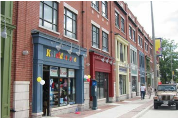
Signage within the entablature framing the shop fronts
