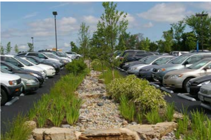
Surface parking incorporating significant landscaping and Low-Impact Development
