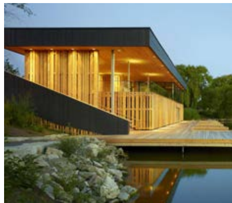
Indigenous Cultural Centre building integrated with waterfront setting (2)
