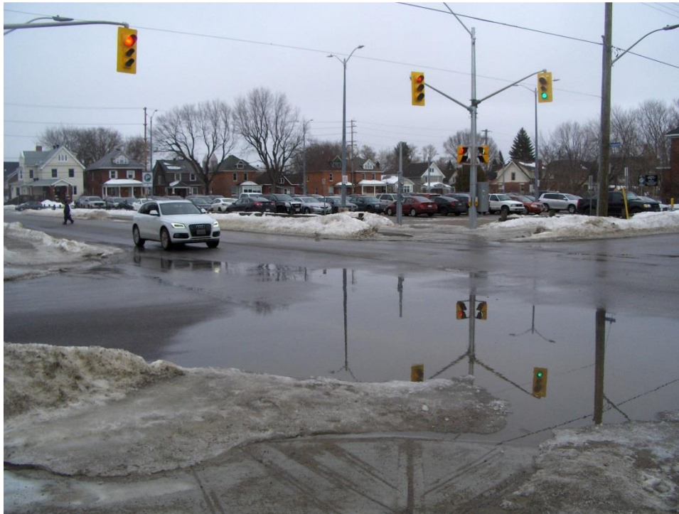
Snow banks and standing water blocking sidewalk access, McIntyre Street
